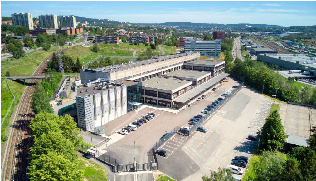
Bulk Data Center, OS-IX (Oslo Internet Exchange)
